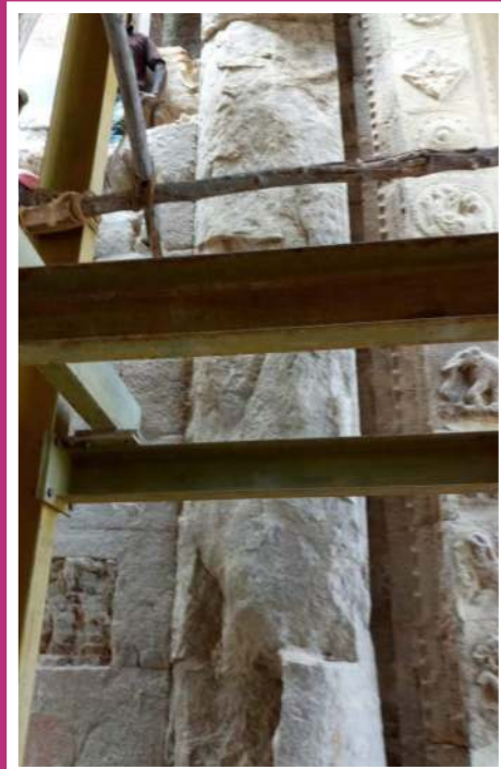
Damaged door frames - Eastern & western side
