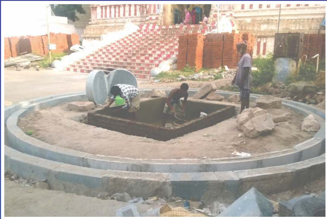
Traditional Lime-Mortar preparing arrangement in construction phase
