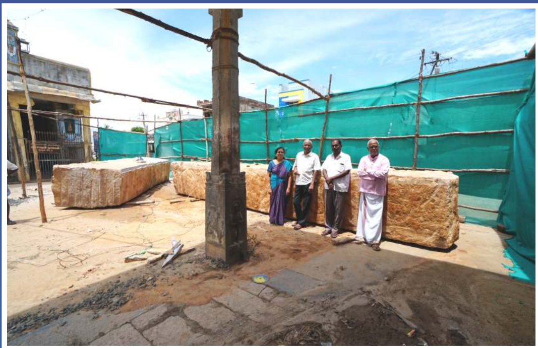
Granite beams arrived from quarry in north of Bangalore August 2017
